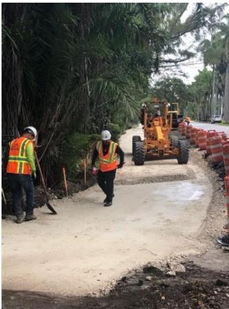
The first phase of the project consists of constructing the shared use path (asphalt) on the East and South sides of the Hollywood Beach Golf Club. This week the contractor, Acosta Tractors, constructed the asphalt foundation for the shared use pathway along 14<sup>th</sup> Avenue from Johnson Street & Polk Street.
